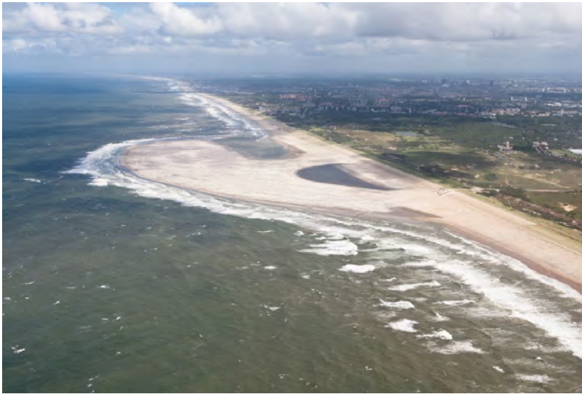
Figure 3.2 Aerial view of the Sand Engine just after completion (9 August 2011 Zandmotor).
